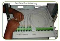
For direct fibre distribution -Arrange the drop cables in circular loops in the patch panel, and then install SC/APC connector. Make sure to clean the before connecting to SC/APC adaptor
