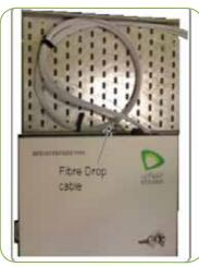
Arrange the cable in the tray in circular loops as shown. Secure the cables using Velcro strap
