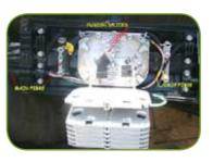
• Pull about 1.5 meters of drop cable into the closure
