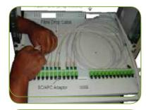
• For direct fibre distribution- Arrange the cable in circular loops in the patch panel, and then install SC/APC connector. Make sure to clean the before connecting to SC/APC adaptor
