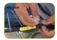
• Install the drop closure cover & fix cable label, and then secure the drop closure in the manhole.
