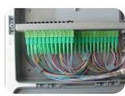
• Connect the fibres in the SC/APC adaptors according to individual port assignments.
