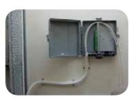
• Install the mini ODF in the designated floor telecom room. Arrange the cable, mark and cut the excess lengths
