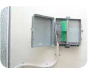
• Re-install the mini ODF in its previous location and provide cable labeling
