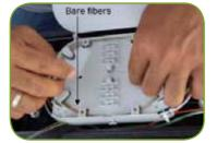
• Arrange the bare fibres in the splice trays, and then close the splice trays
