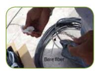
• Remove the protective tubes and clean the bare fibre using alcohol
