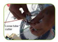
• Cut the protective tubes using loose tube cutter
