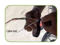
• Wrap the cable end using electrical tape
