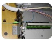
• Remove the cable outer sheath and prepare individual fibres for connector installation
