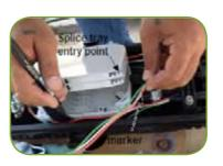
• Route the loose tubes in the splice tray entry point and mark
