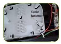
Route the fibre in the splice tray and secure the protective tube using cable fastener
