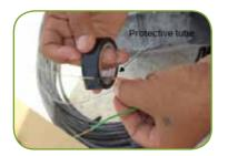
• Wrap each protective tube's end using electrical tape
